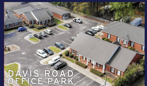
DAVIS ROAD OFFICE PARK UP TO 1600 SF
