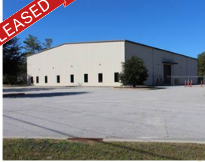
3831 WRIGHTSBORO ROAD TENANT REP - INDUSTRIAL 12,000 SQUARE FEET
